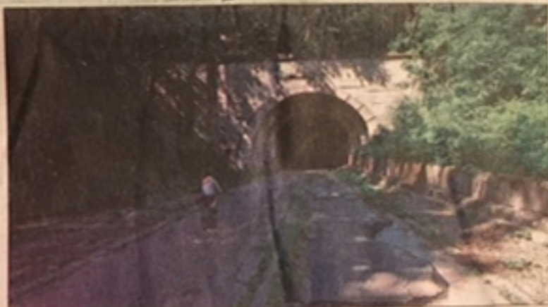
This photo was taken at the Sideling Hill Tunnel shortly after the area was cleared by the Old PA Pike Trail Committee.
